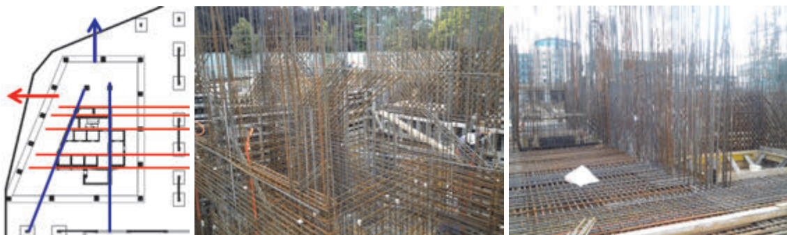
Fig. 9: Tower B layout, diagonal reinforcement of the walls and ground floor slab reinforcement
