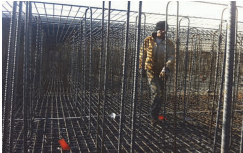
Fig. 4: The 2.00 m slab with the traditional reinforcement
