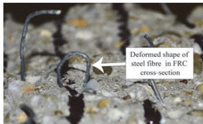
Fig. 6: Deformed shape of steel fibre in cross-section of beam by the 30 min mixed SFRC
