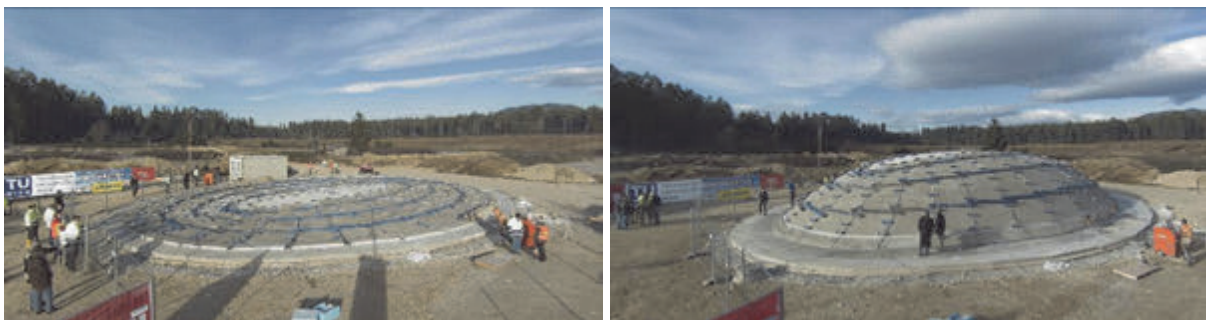
Fig. 11: Initially flat plate (left) and finished concrete shell (right) (© webcam of Dipl.-Ing. Wolfgang Reinisch - http://reinisch.at/ on behalf of the Austrian railways (ÖBB))
