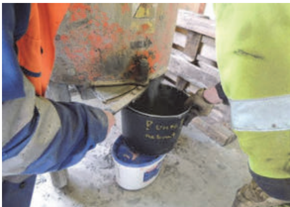
Fig. 4: Fresh UHPC poured into a bucket Fig. 5: Fresh UHPC poured into a form
