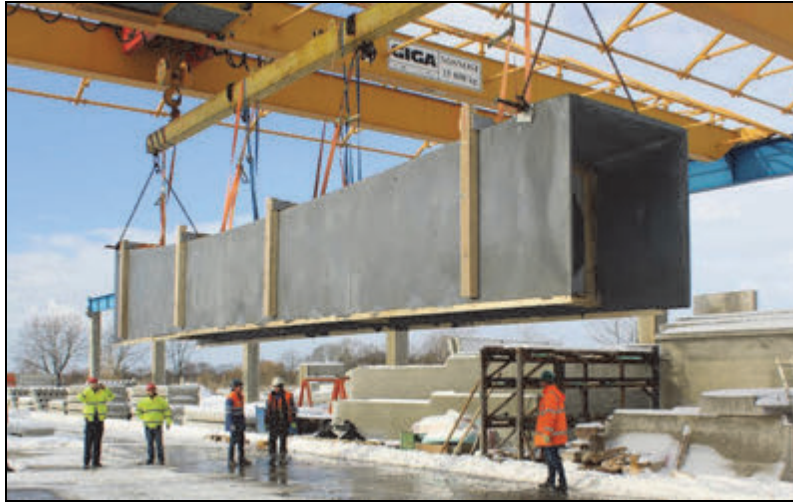
Fig. 10: Transport of final 1:1 mock-up of the footbridge in upside-down position
