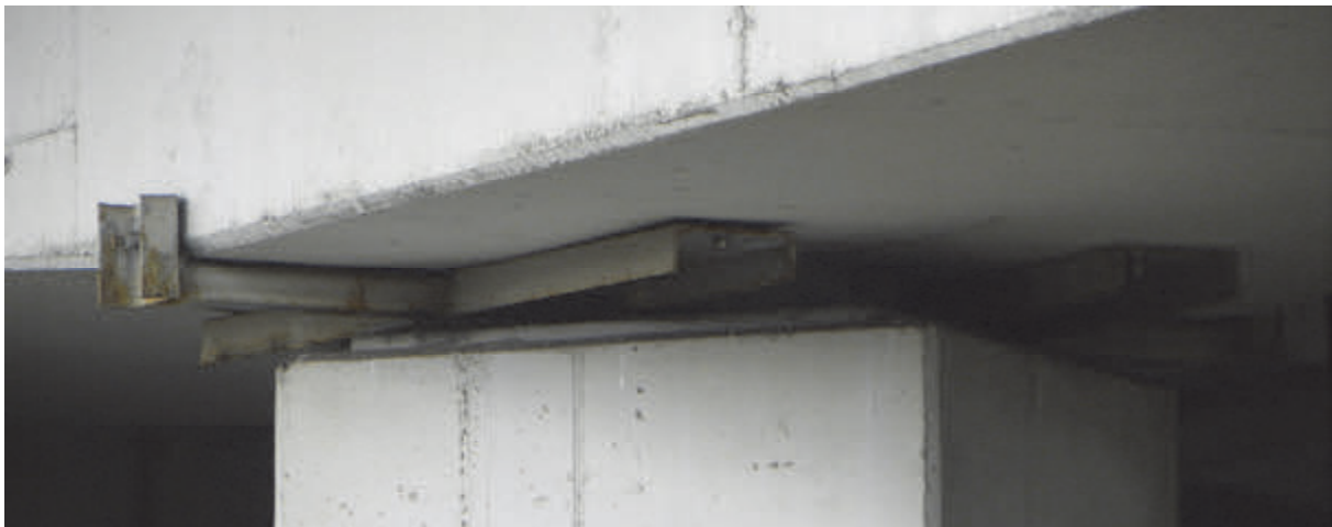
Fig. 8: Stabilisation of displacement direction of chamfered fixed bearing
