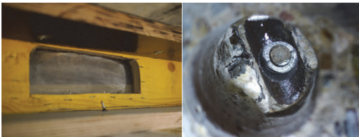
Fig. 4: Observation window with Perspex cover (left) and severed prestressing tendon at deactivation drill hole (right)
