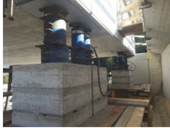
Fig. 8: Lowering stack
