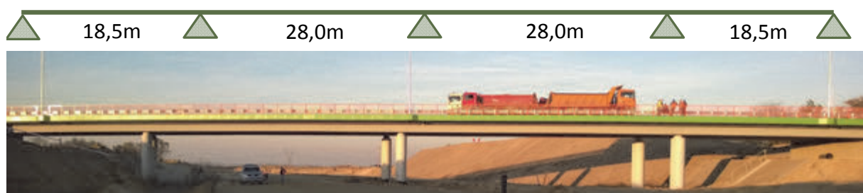
Fig. 1: Static scheme and view on bridge WD-247 (A1 motorway; section Stryków - Tuszyn)
