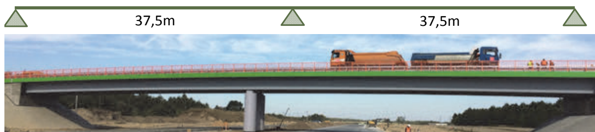
Fig. 2: Static scheme and view on bridge WD-267 (A1 motorway; section Stryków-Tuszyn)
