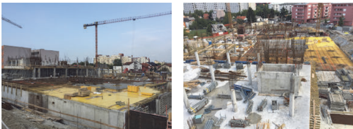
Fig. 22: J12 building under construction
