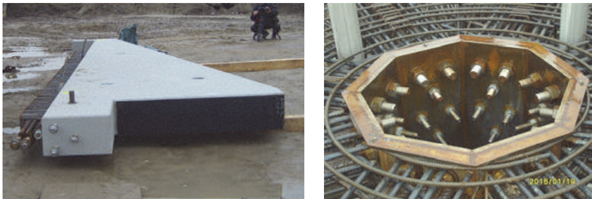
Fig. 3: Anchoring of cantilevers to the final mast element (Type 2)
