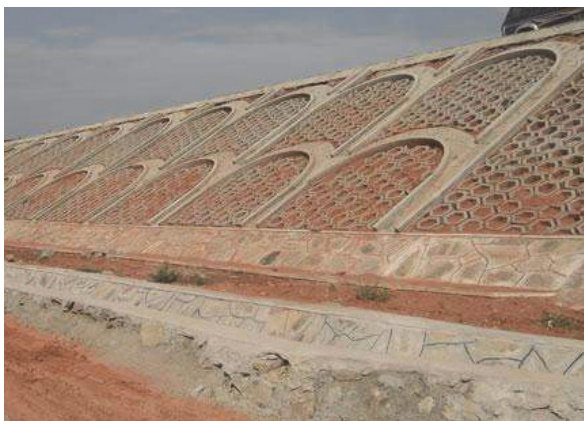
Fig. 5: Highway bank protection revetment
