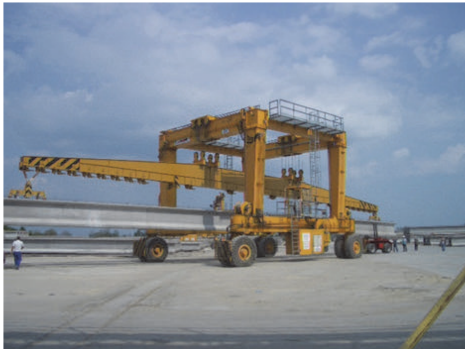
Fig. 5: Transportation of bridge girders within the Dunaújváros plant
