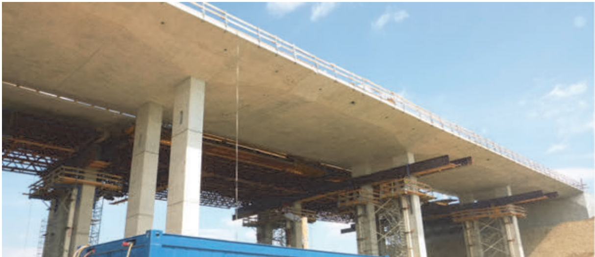
Fig. 3: View of the superstructure from below
