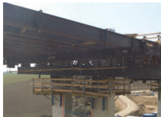
Fig. 8: Temporary support of the scaffolding and formwork of the new superstructure segment on the previous superstructure segment (left) and piers (right)
