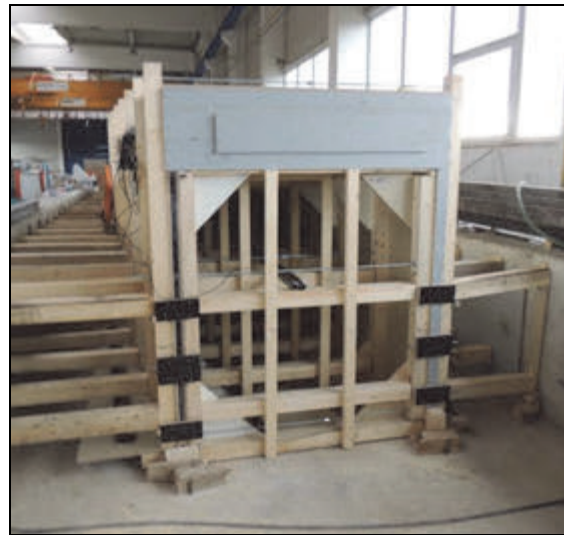
Fig. 9: Formwork prepared for the casting
