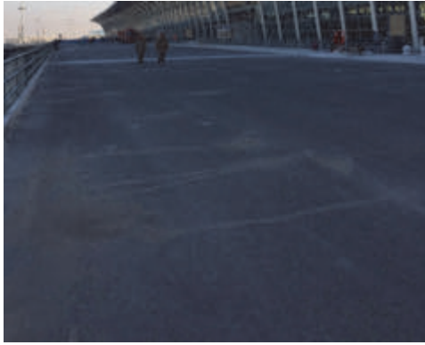
(a) A prestressed concrete bridge
