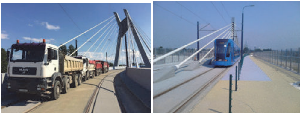
Fig. 7: Static and dynamic tests
