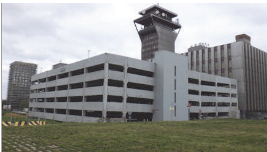
Fig. 2: The finished structure with apparently inclined floors
