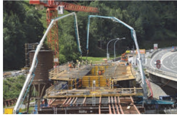
Fig. 5: Concreting of section 1 superstructure
