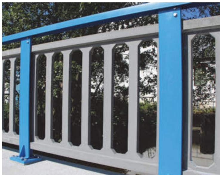
Fig. 6: Detailed view on the UHPC railing panel on the bridge in Sázava
