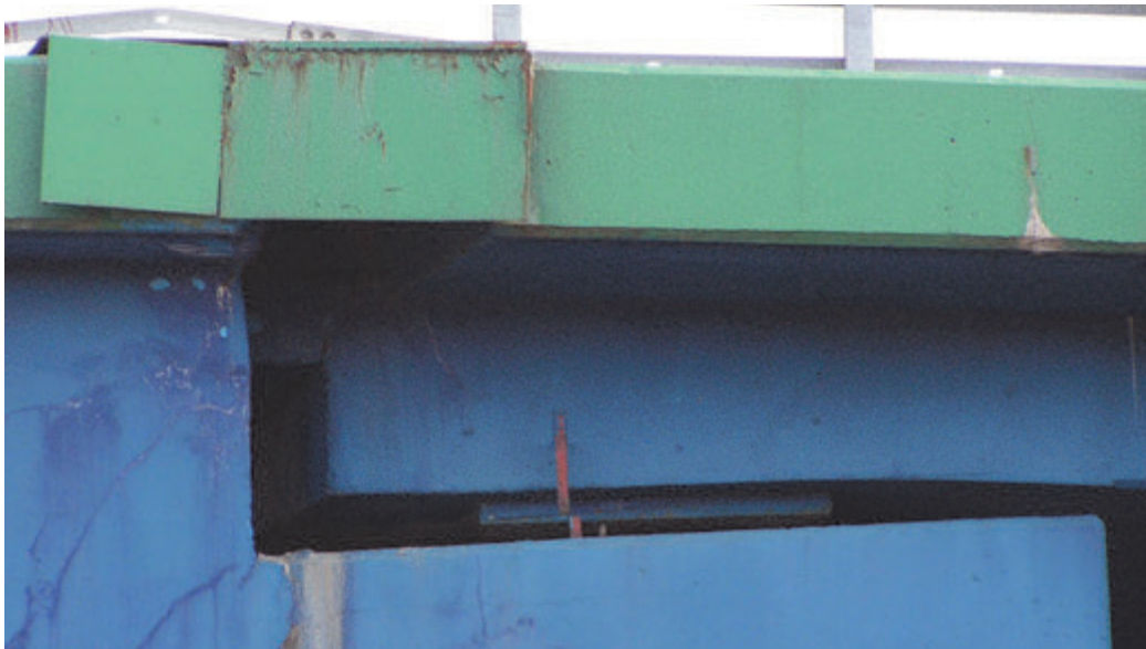
Fig. 3: Connecting the structure with embankment by means of an approach slab
