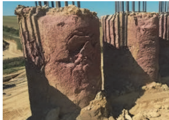
Executed piles – earth dam partly removed
