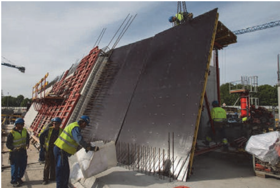
Fig. 6: Museum of the Second World War under construction. pict. R. Jocher
