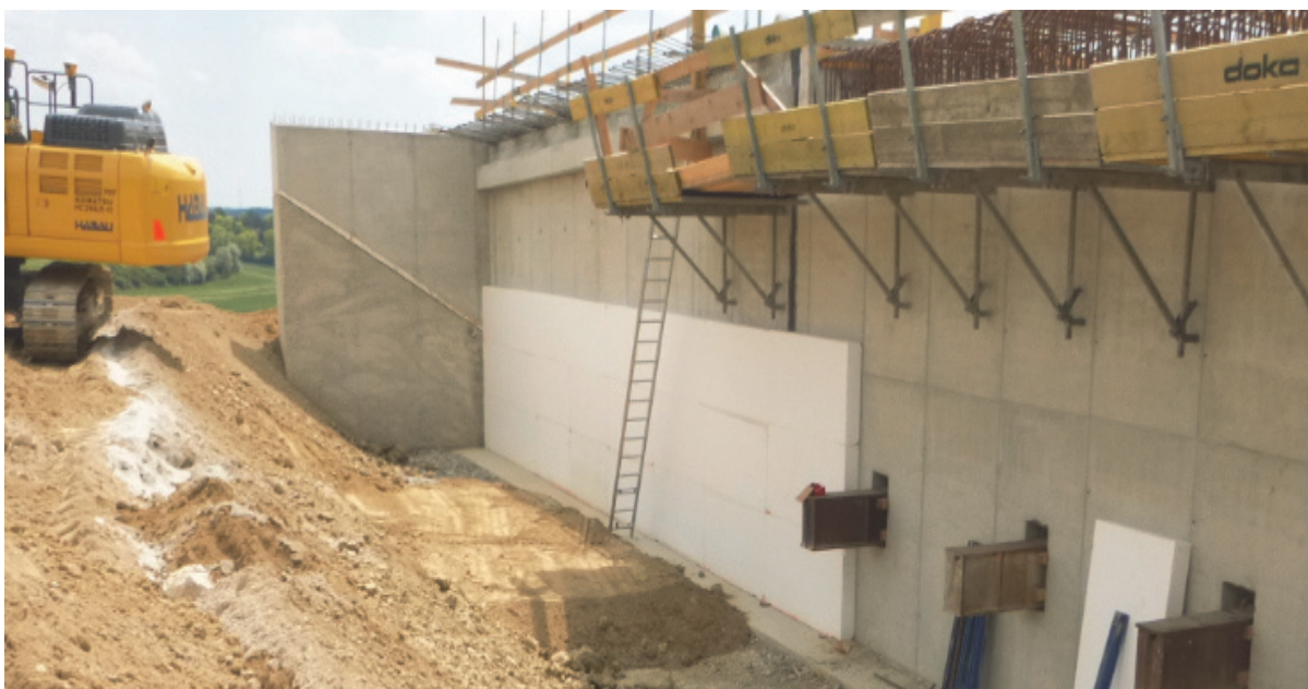
Fig. 5: EPS on the back of the abutment wall
