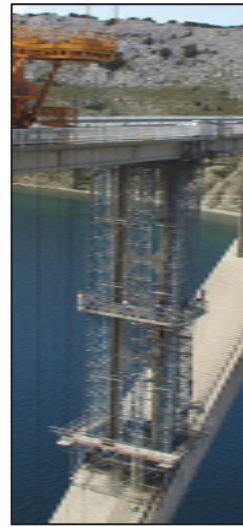
Fig. 5: Disburdening of the column S 26
