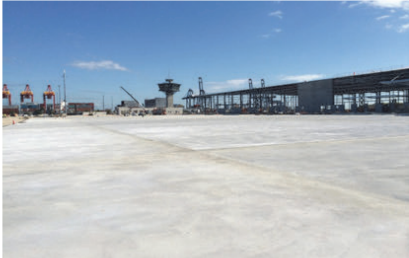
Fig. 1: 50,000 m 2 seamless slab with hybrid reinforcement
