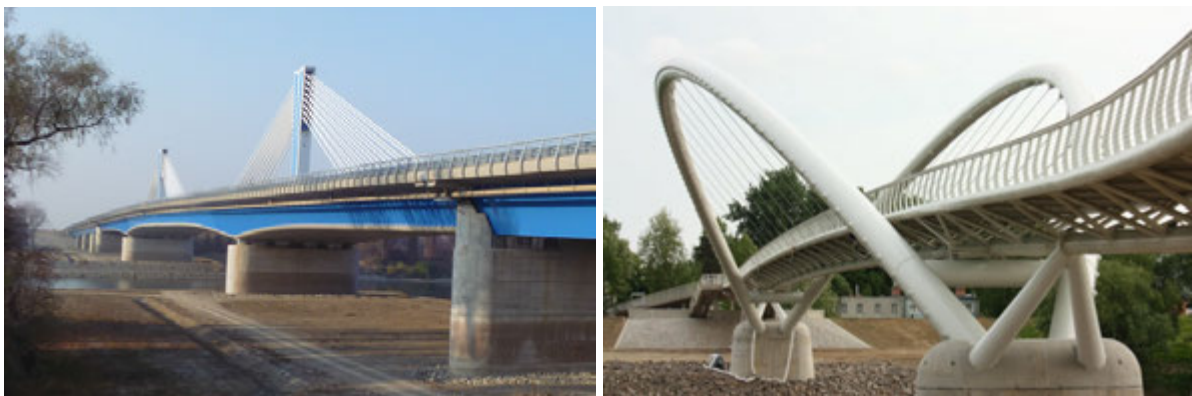
Fig. 5: The most unique bridges over the river Tisza
