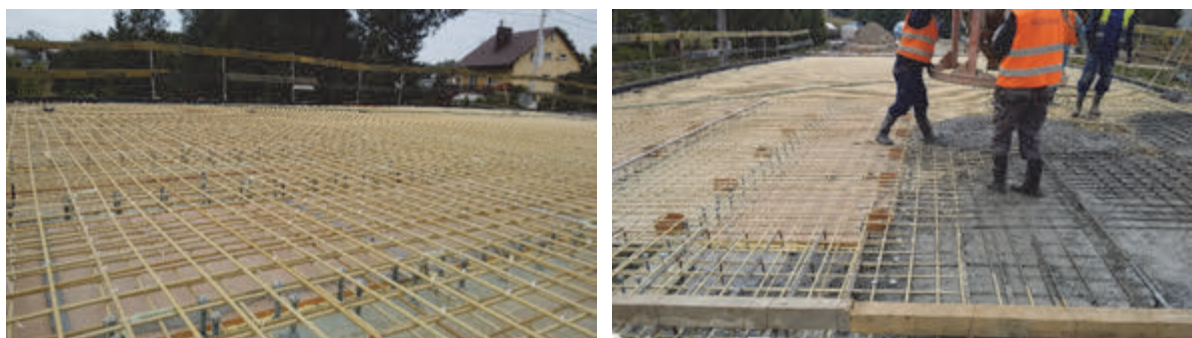
Fig. 8: Installation and construction of a lightweight concrete bridge deck slab reinforced with GFRP rebars
