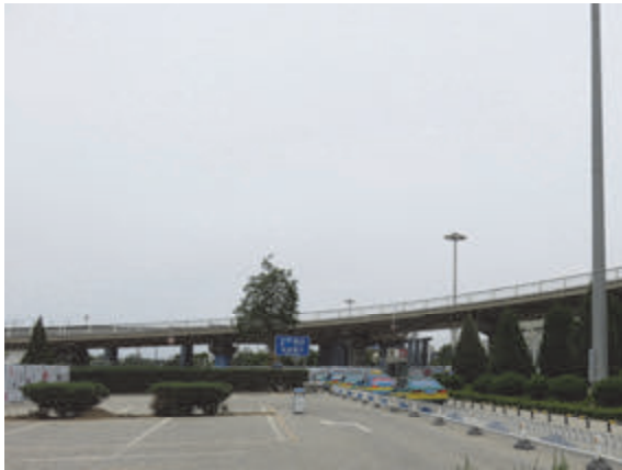
(a) A concrete bridge to be demolished
