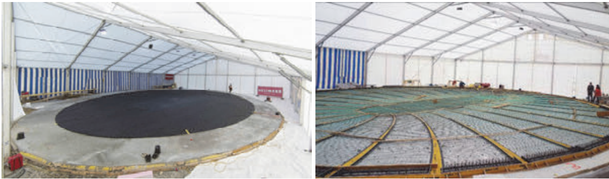
Fig. 10: Air cushion (left) and ready mounted reinforcement of the flat plate (right)
