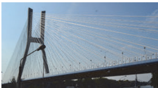
Fig. 2: View on Rędziński Bridge in Wrocław
