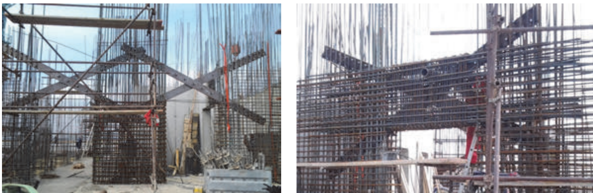
Fig. 7: Coupling beam with diagonal steel plates
