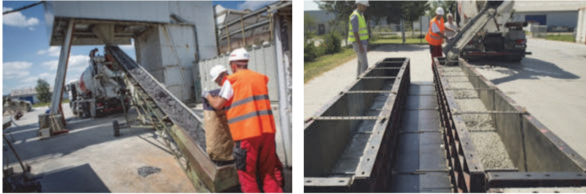
Fig. 3: Fiber addition via conveyor belt (left) and filling of the beam from one side (right)
