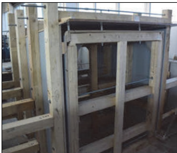
Fig. 2: Formwork of the preliminary mock-up
