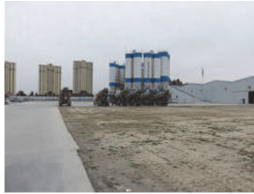
(b) A precast concrete plant
