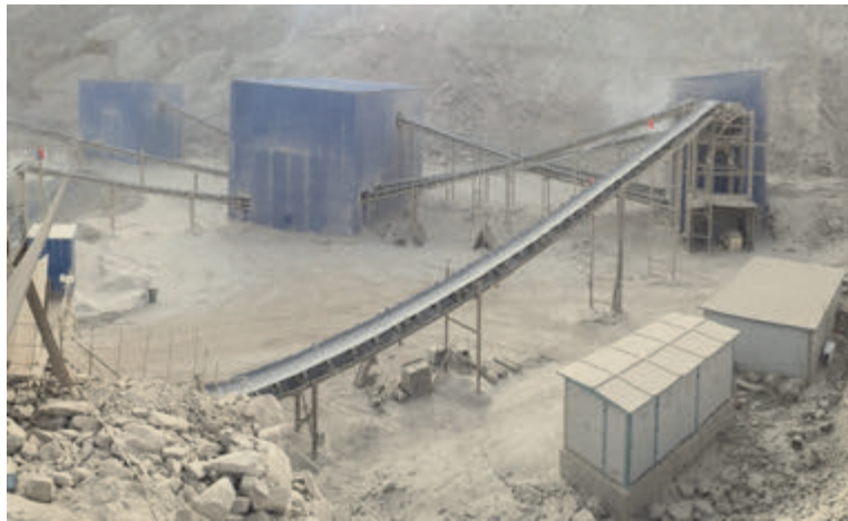
Fig. 2: Crushing plant for concrete aggregates
