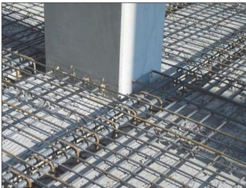
Fig. 5: View of prefabricated structures and reinforcement before concreting floors
