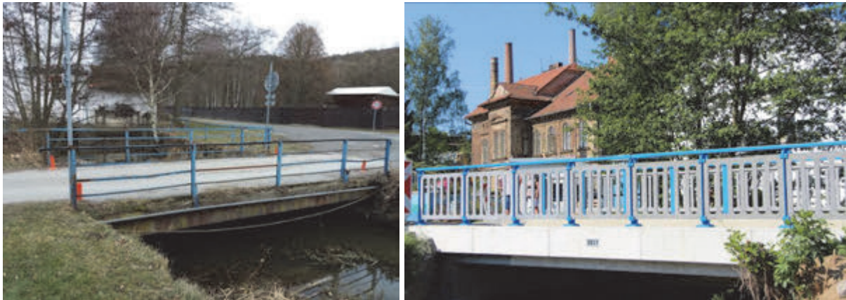
Fig. 7: Comparison of the bridge in Sázava before / after the renovation
