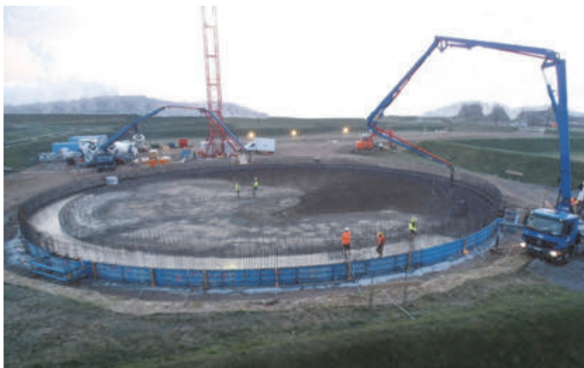
Fig. 2: Pouring of the liquid tight raft foundation
