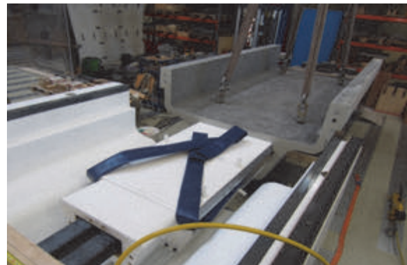
Fig. 9: Formwork / QUICKWAY Segment
