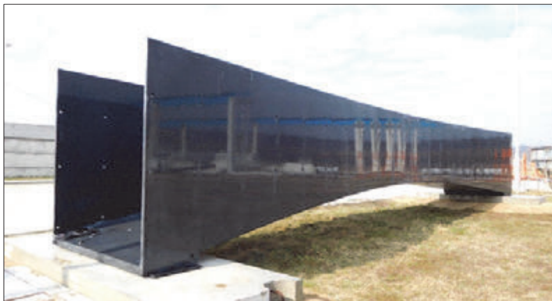
Fig. 11: Storing of the footbridge in correct position
