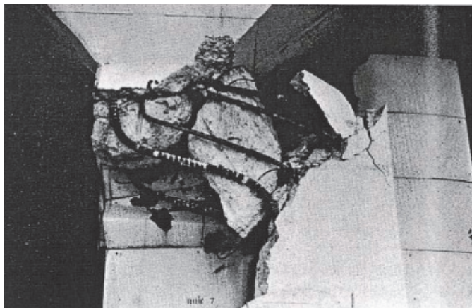
Fig. 7: Example of a shear failure in an unexposed concrete column due to the thermal expansion of the fire exposed floor connected to it (Beitel and Iwankiw, 2002)
