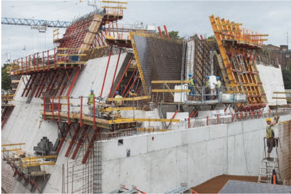
Fig. 7: Museum of the Second World War under construction. pict. R. Jocher
