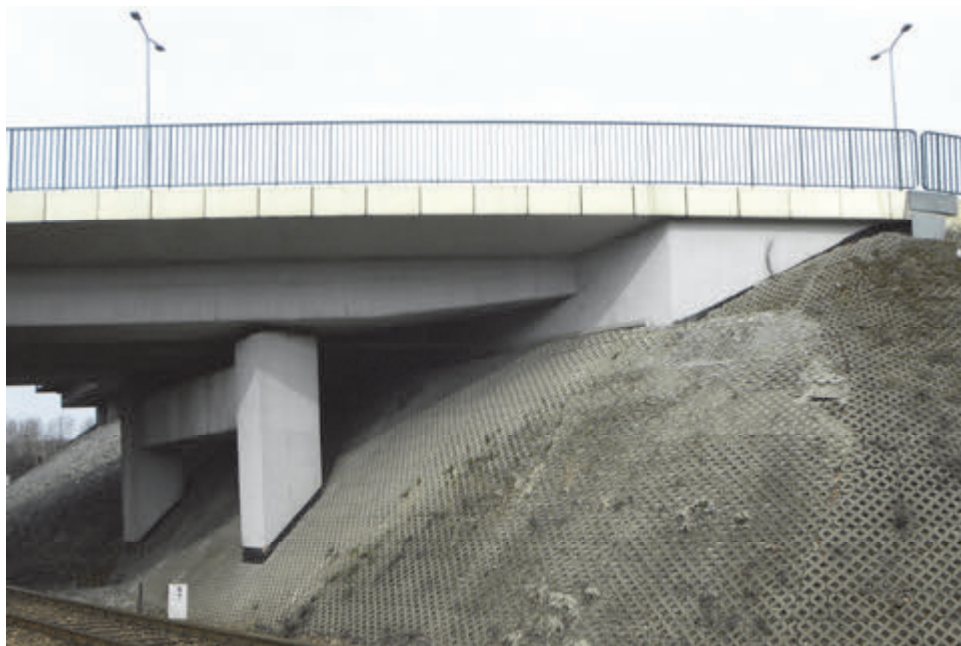
Fig. 6: Exemplary solution of the load-carrying structure with cantilevers
