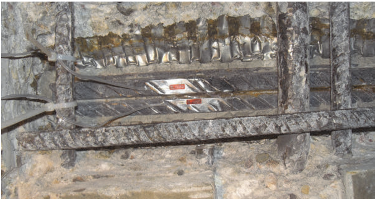
Fig. 5: Strain gauges mounted on the ribbed prestressing cables
