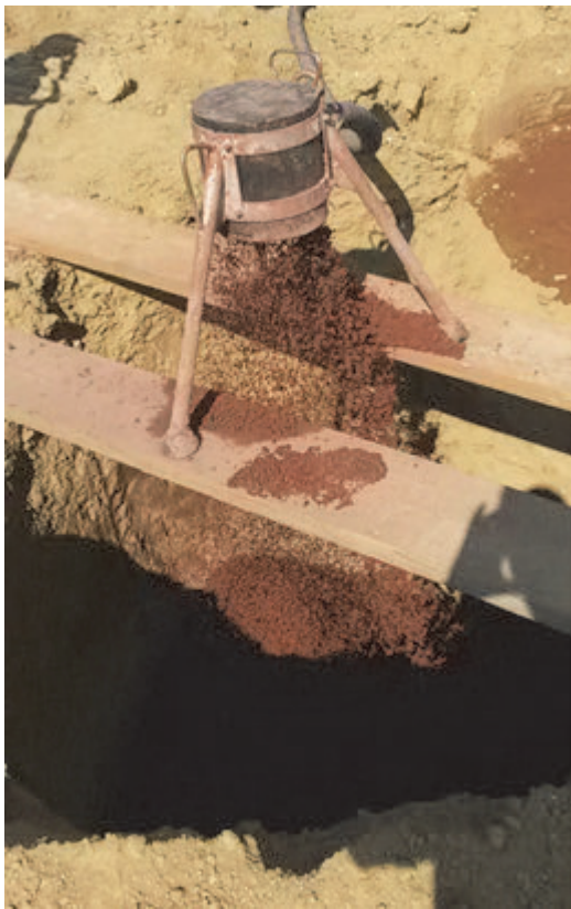
Filling of the 1.8 m bore hole with the polystyrene granulate cement mixture
