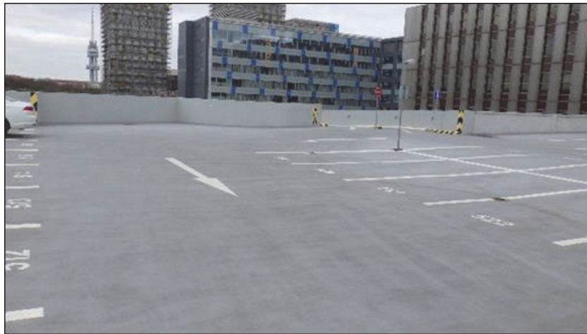
Fig. 6: Roof of garage with the parking floor after five years of service
