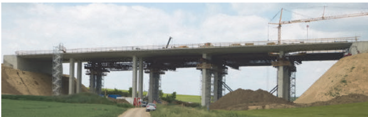
Fig. 1: View of the bridge
