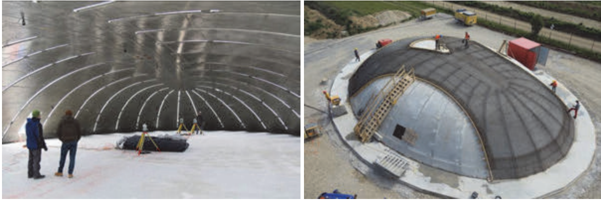
Fig. 12: View from inside of the shell for the event canopy after inflation (left) and ready mounted reinforcement for the additional concrete layer
