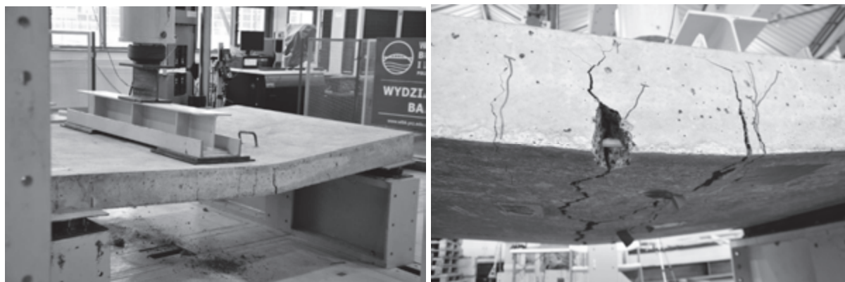
Fig. 6: Slab failure pattern after the fatigue test
