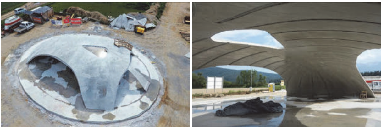
Fig. 13: Event canopy during the cutting process with view from above (left) and view from inside (right)
