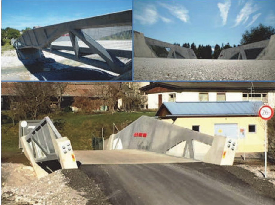
Fig. 11: Paulifurt bridge in Carinthia in Austria
