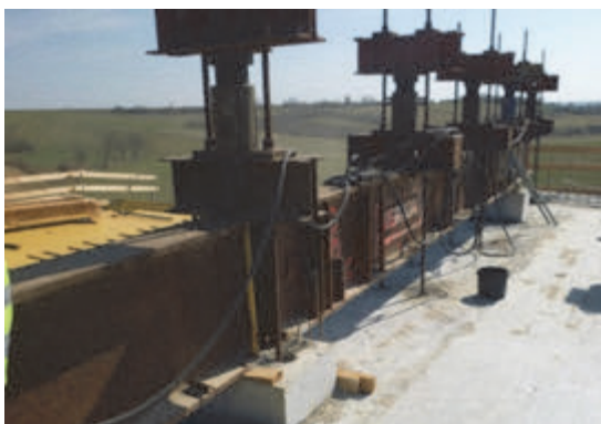
Fig. 8: Temporary support of the scaffolding and formwork of the new superstructure segment on the previous superstructure segment (left) and piers (right)
