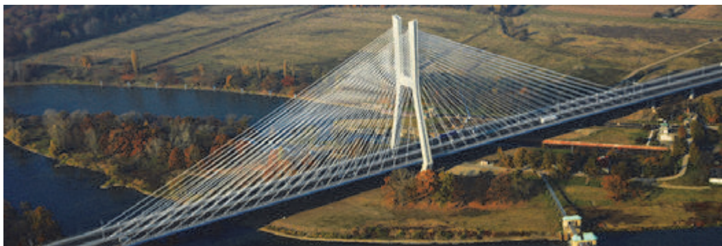
Fig. 1: View of the Rędziński Bridge [ www.golowersilesia.pl ]
