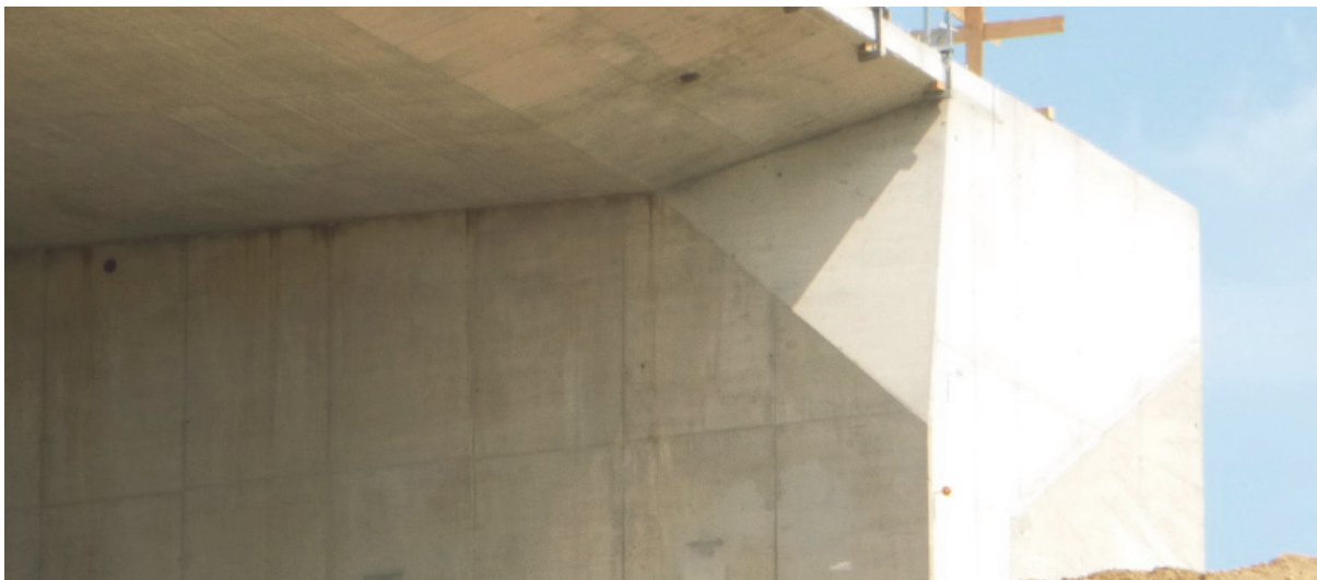
Fig. 4: Detail of the abutment wall
