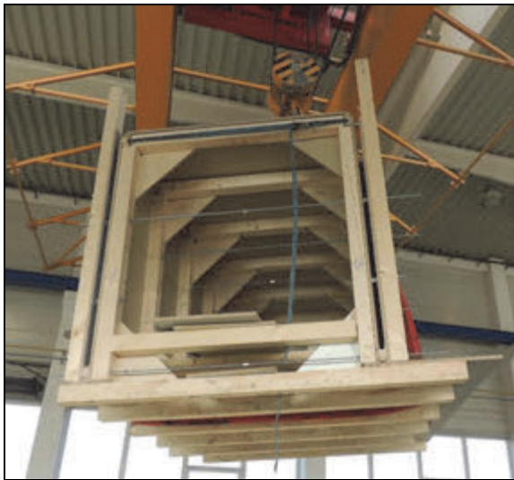
Fig. 8: Transport of the 1/4 of the formwork
